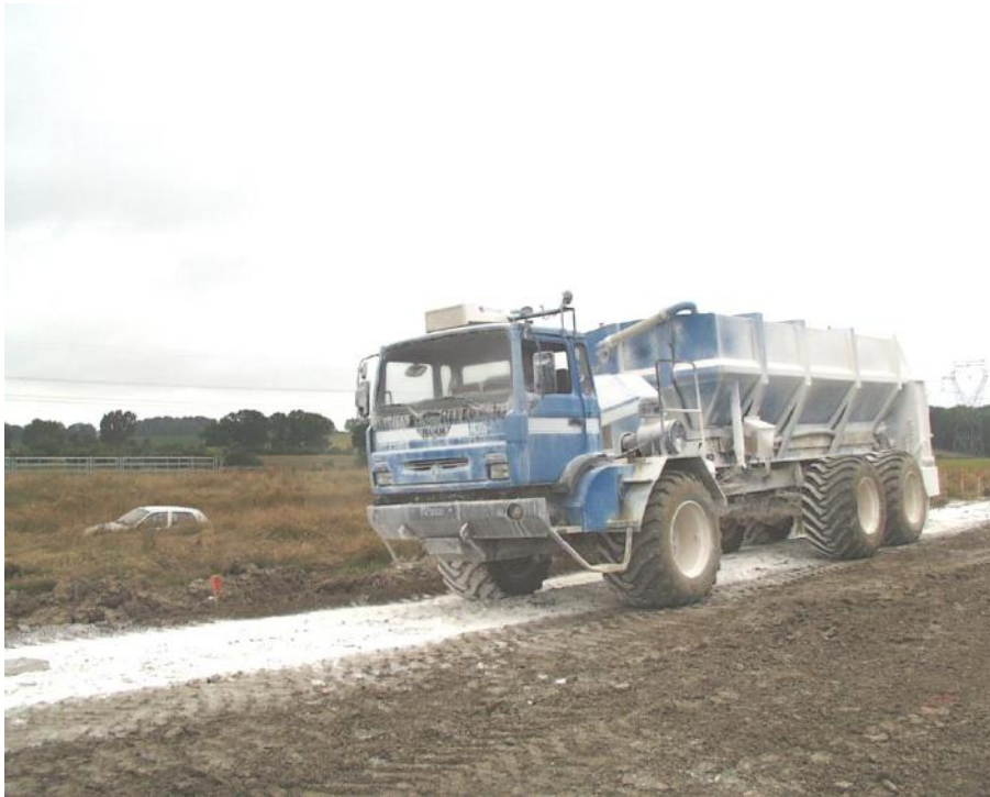
Treatment in the embankment
