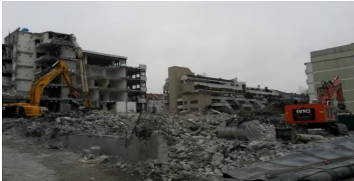
selective deconstruction of buildings and roads
